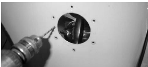
Figure 149: Carefully drill new holes
