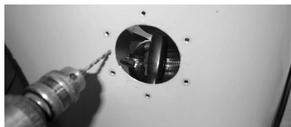
Figure 186: Carefully drill new holes
